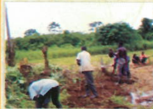
Fig. 3: Remove tree roots and stumps
