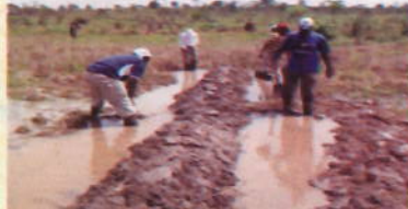
Fig. 5: A bund under construction
