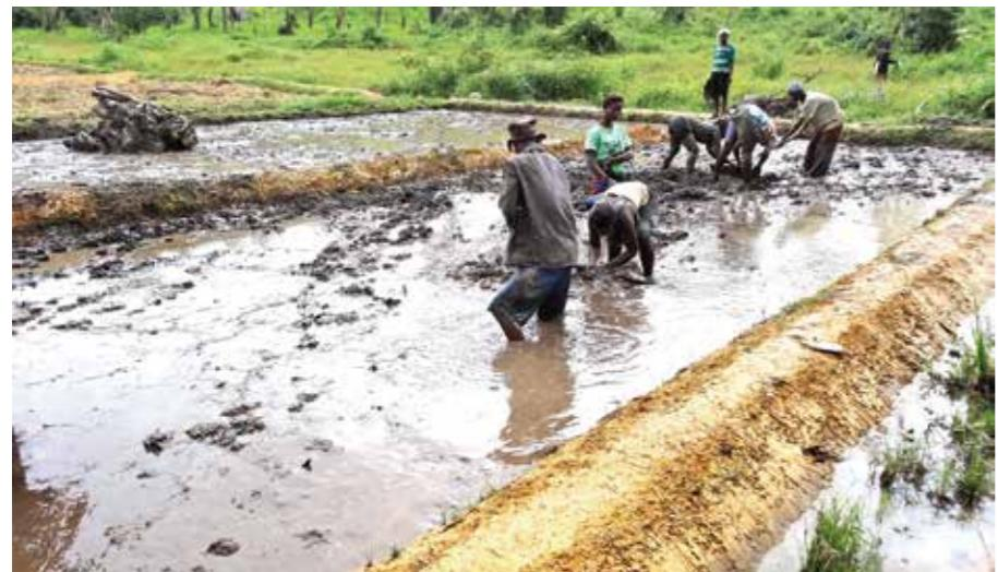
Fig. 26 Inner Bonds and levelling
