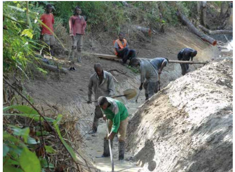
Fig. 20a Peripheral floodway in Bettijama
