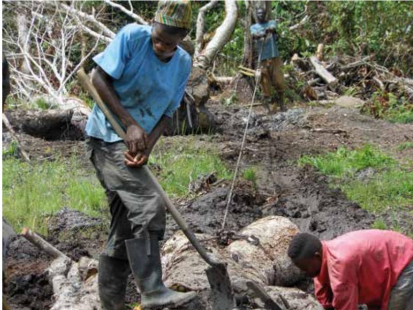
Fig. 18 De-stumping Abura tree with the help of cable pulling device "Come Along"
