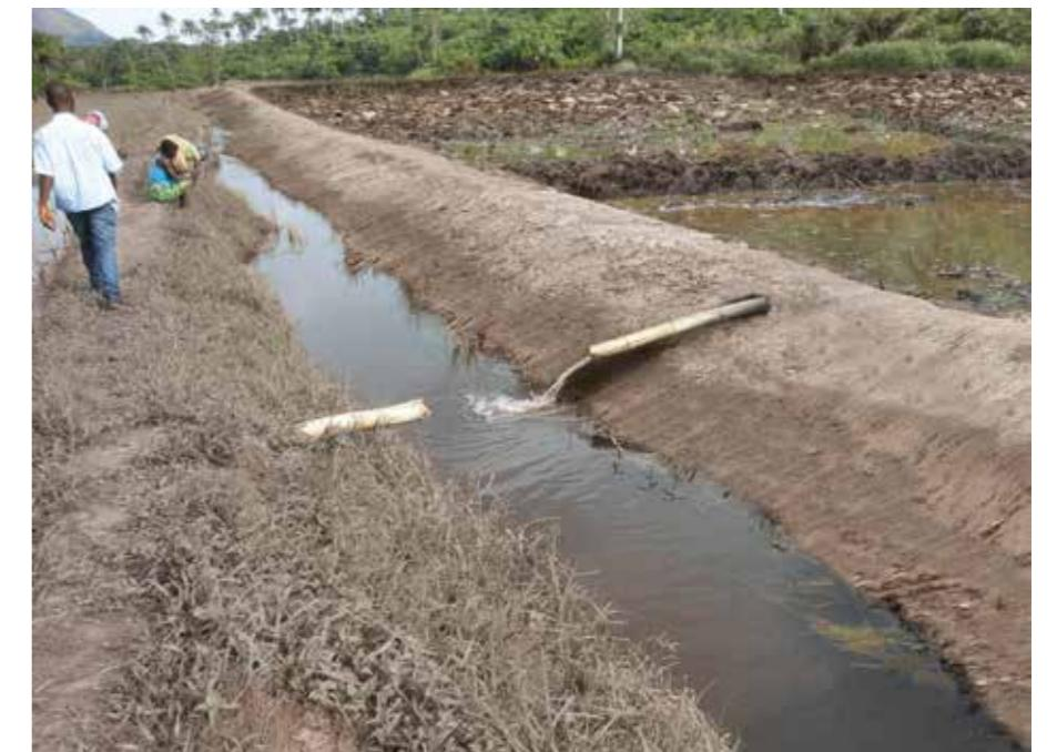
Fig. 28 Bamboo or PVC Pipe per plot for drainage
