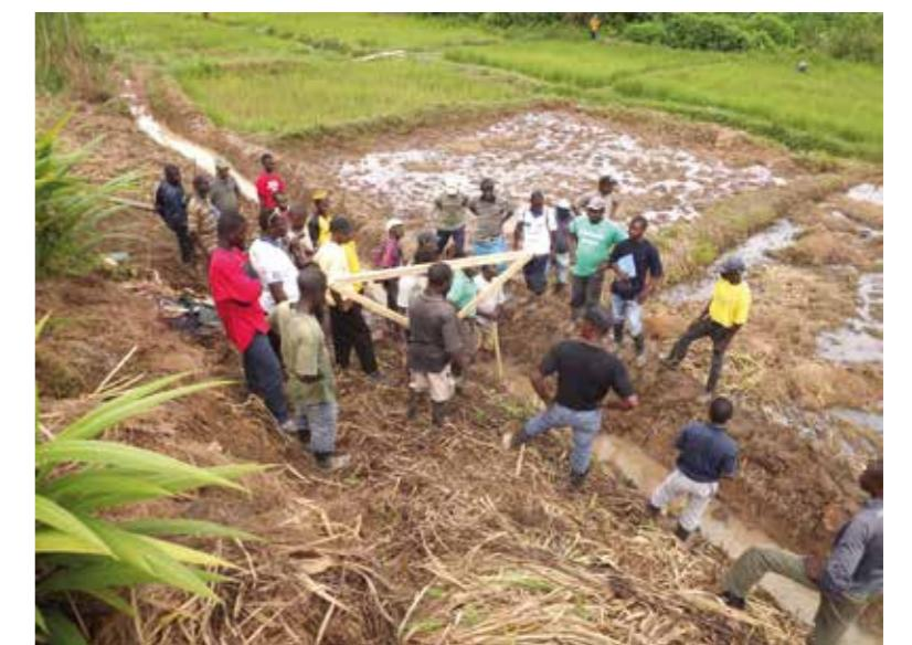
Fig. 25 Using Model for Shaping Peripheral Canal and Dimensions of Supply Canals
