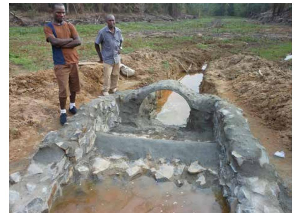
Fig. 23a Dig form-work in compacted soil, both ends 100 cm deep in ground. Arrange space for headpan to empty groundwater. Place good quality stones well tied together.
