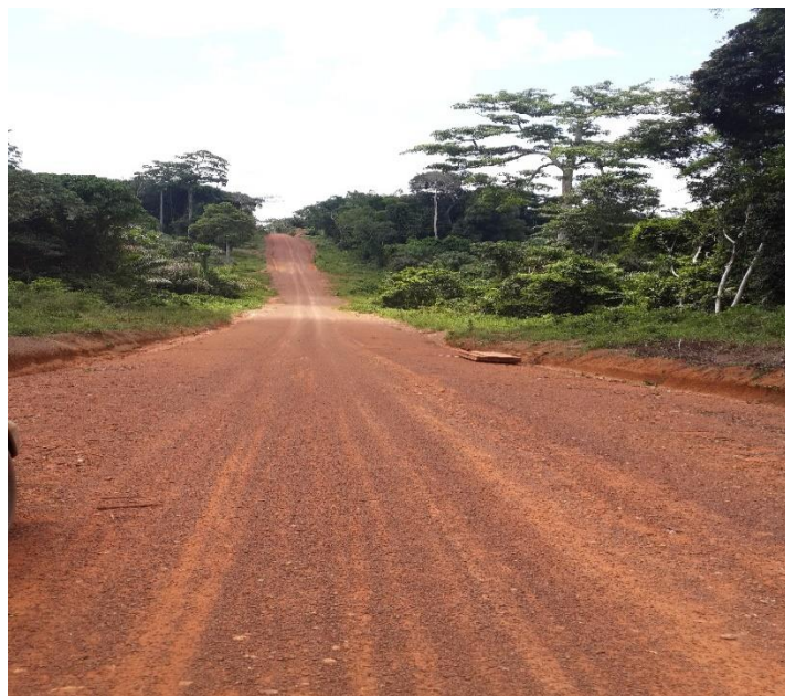
Photo 2: After Construction of 27KM Zwedru-Ziah Town Road in Zwedru, Grand Gedeh County
