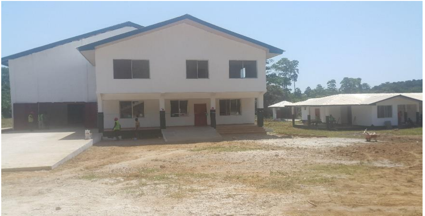
Completed Processing/milling and Management facilities ready for dedication and handover
