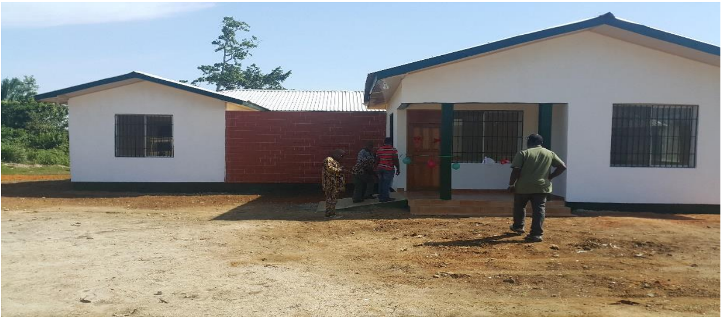
Completed MoA Office ready for dedication and handover
