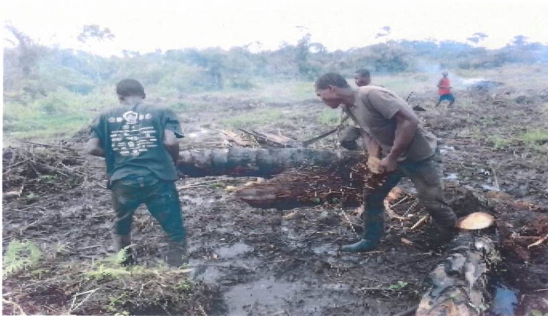
Land clearing and debris removal after burning
