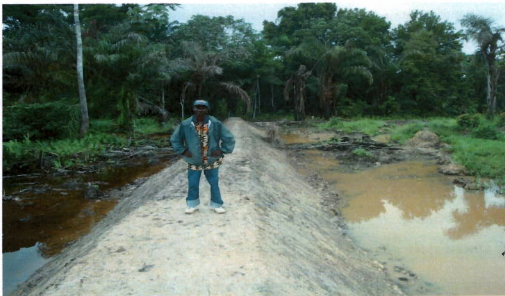
Constructed head dyke
