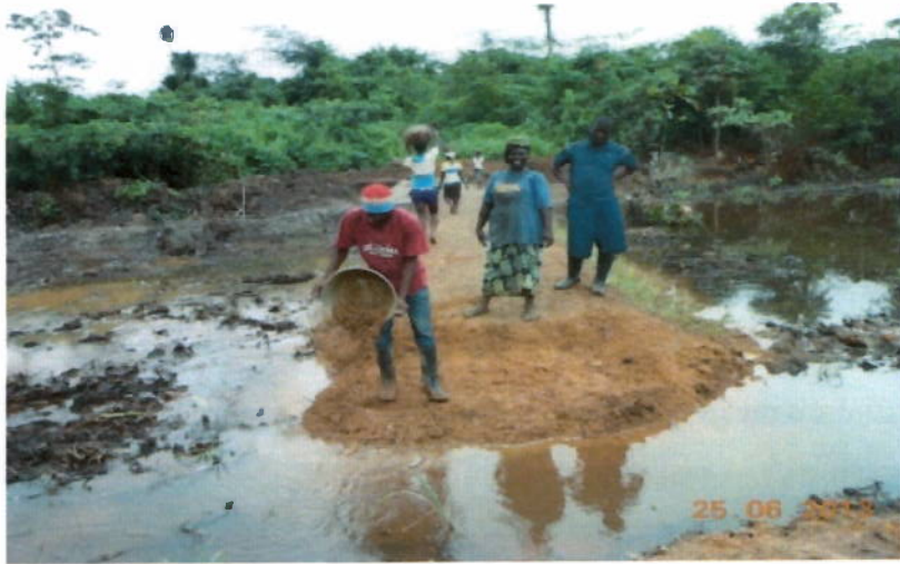
Head dyke under construction
