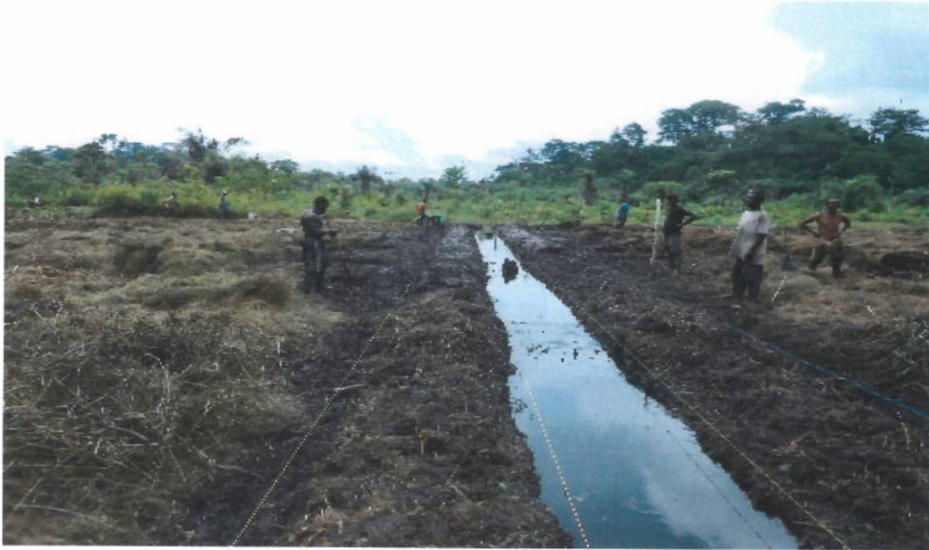
Pegging, layout, canal and bund construction
